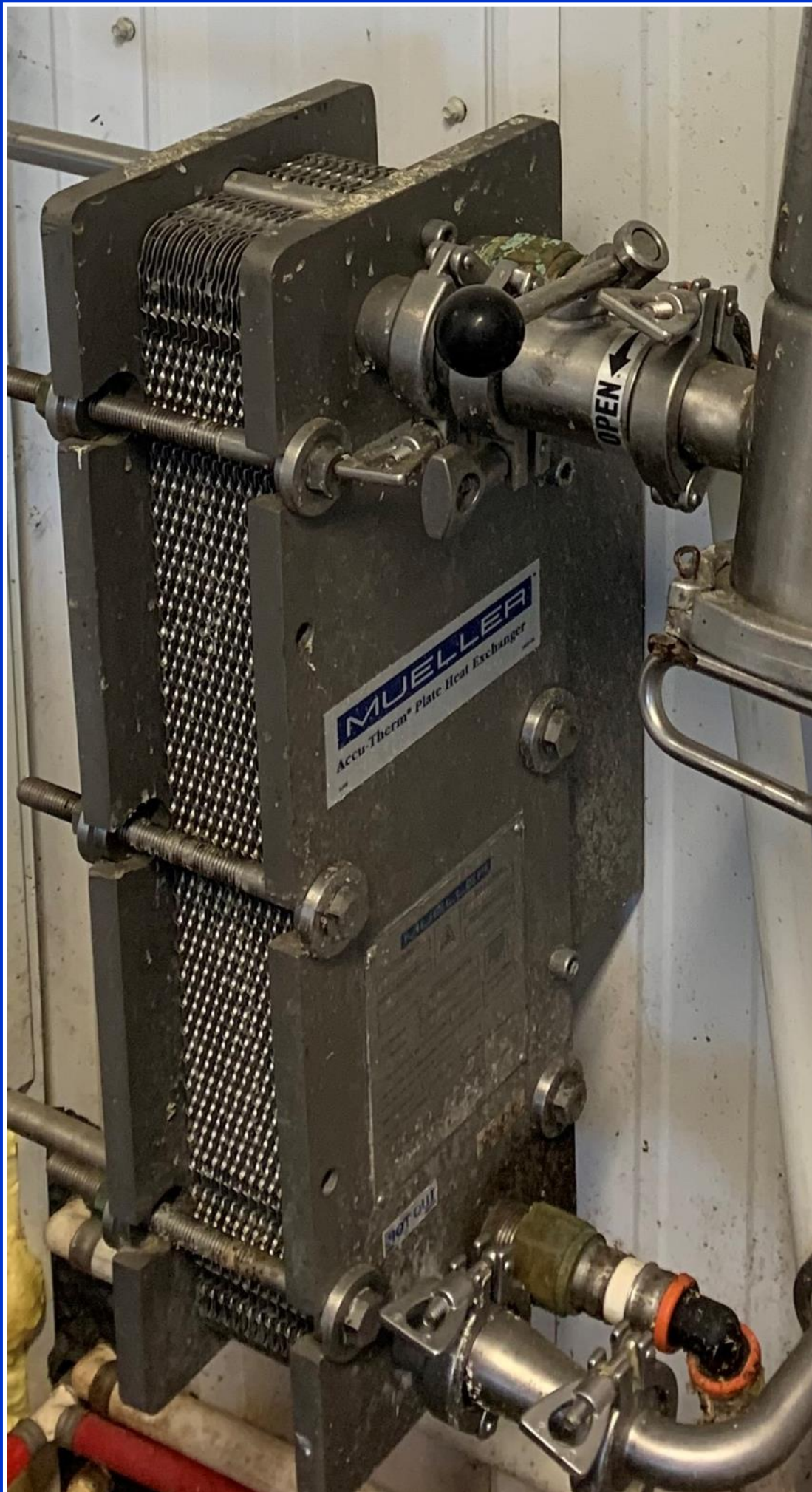
Mueller Plate Cooler Model: AT4 DW-31 Serial #: 143720 Plates: 31
